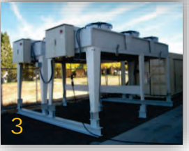
Small Scale Power Generation from Co-Produced Geothermal Fluid - Electratherm has successfully demonstrated the technical and economic feasibility of geothermal energy production through a state-of-the-art Organic Rankine Cycle (ORC) heat-to-power generator.
