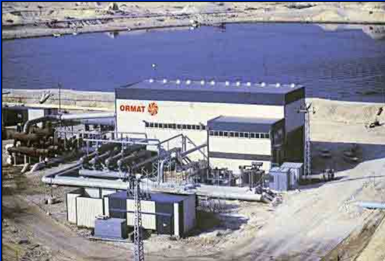
5 MW Solar Pond Collects and Stores Energy - 1982
