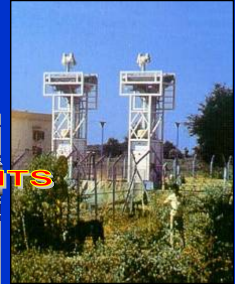
HBJ Gas Pipeline Project, India
