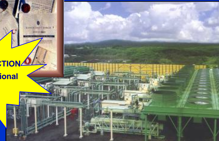
Puna Geothermal Power Plant, Hawaii
