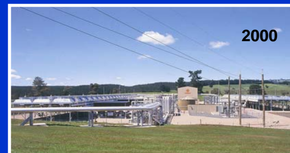
60 MW Mokai Combined Geo'mel Power Plant, New Zealand
