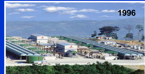
125 MW Upper Mahiao Combined Geo- Power Plant, Philippines
