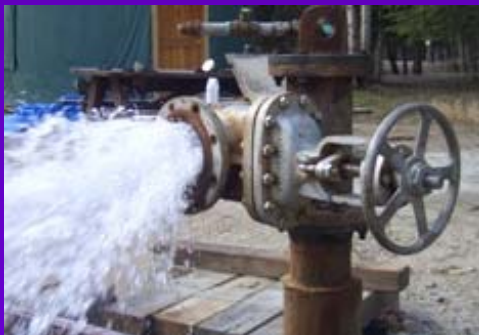
Geothermal Wells Provide Hot Water (~165F)
