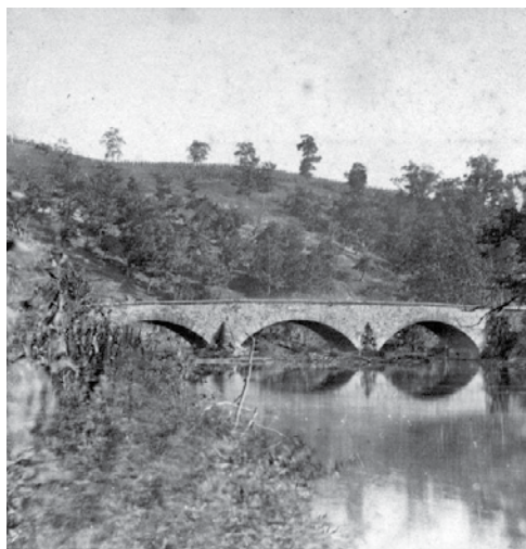
"Antietam Bridge. Looking down stream," September 1862, albumen stereograph, by Alexander Gardner. Courtesy of the DeGolyer Library, SMU.
