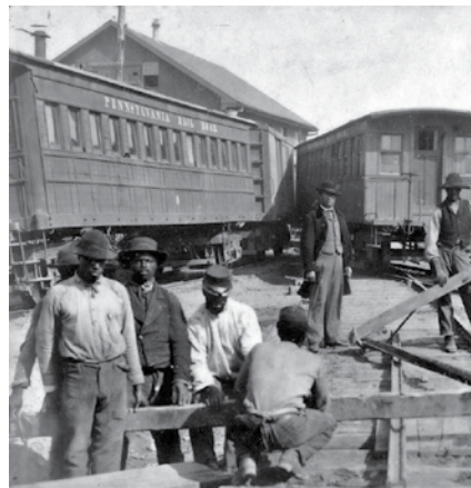
“Military railroad operations in northern Virginia: men using levers for loosening rails,” ca. 1862-1863, salt print, by Andrew J. Russell. Courtesy of the DeGolyer Library, SMU.
