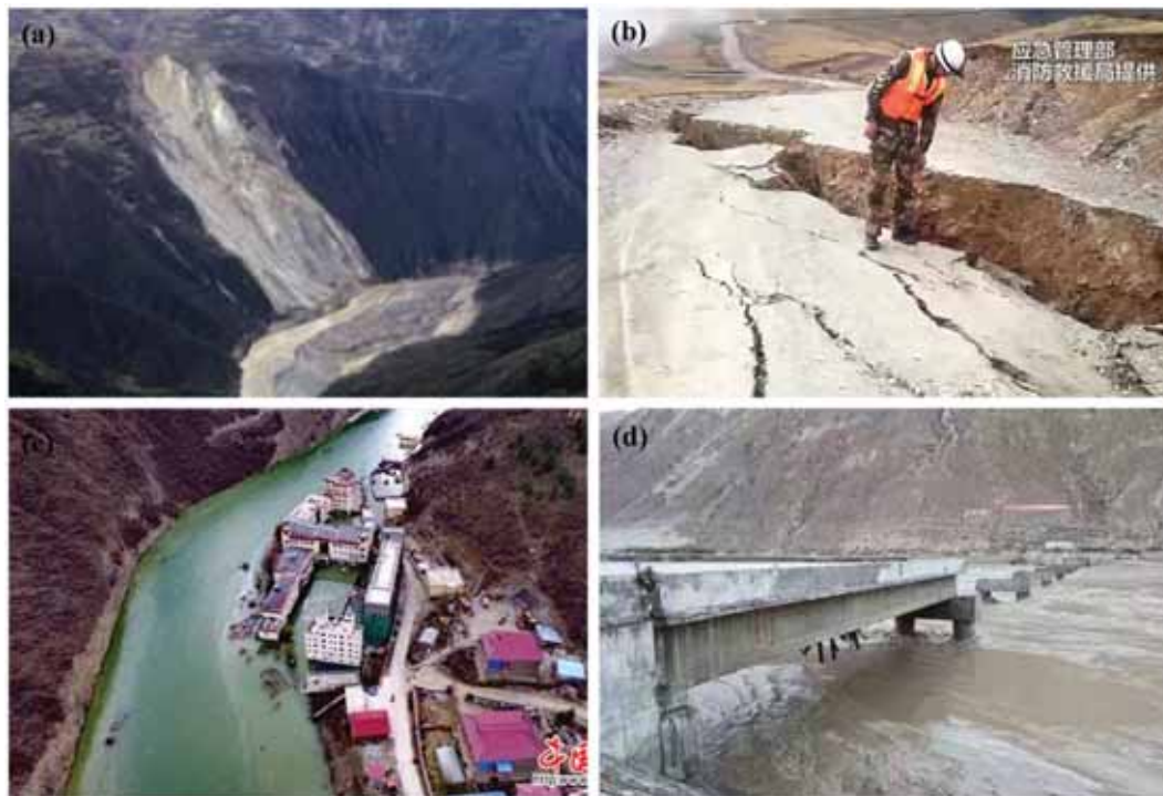
Fig. 2. The case of the Baige landslide, Jinsha River (source: https://image.baidu.com/ ). (a) View after the occurrence of the landslide on October 11, 2018; (b) road damage; (c) flooded houses; and (d) bridge damage.
