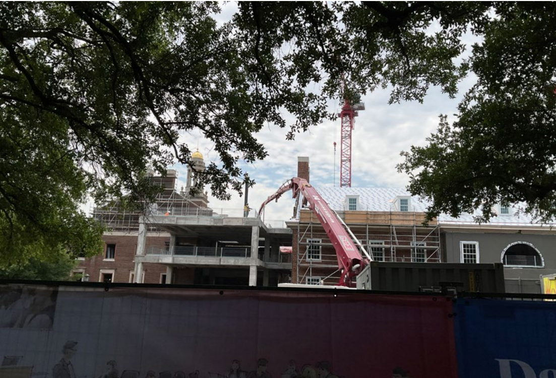
This photo captures the final elevated concrete pour at Shaddock Hall.
