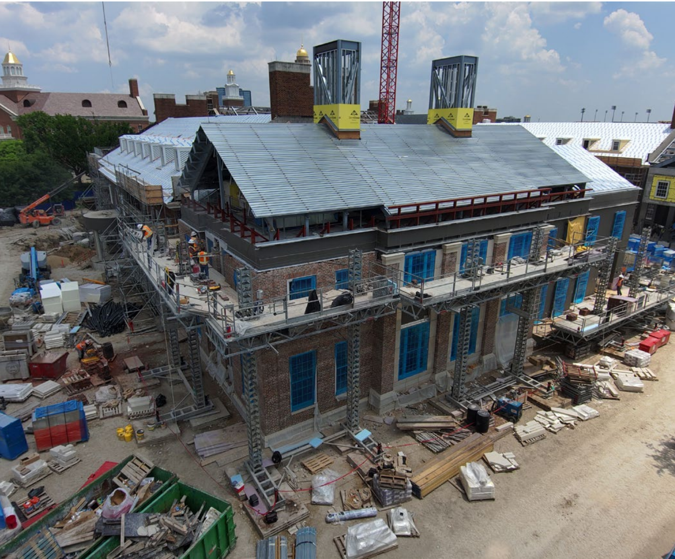
By mid-June, brick covers much of the exterior of Bolin-Bridwell Hall.
