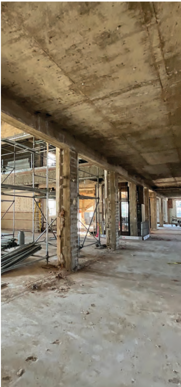
Down to the studs in the Fincher Building hallway. This is the view just outside the EY Gallery.
