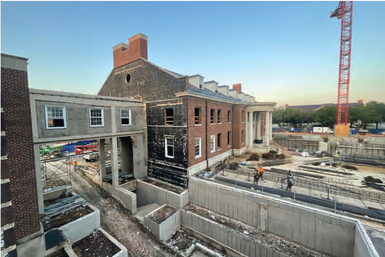
The “bridge” that connected the Fincher Building to the Crow Building, and the columns and stairs beneath, are on the way to being demolished in this photo, taken mid-summer.
