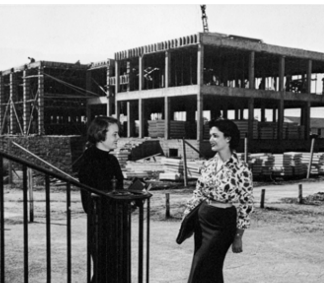
The Fincher Building under construction in 1953
