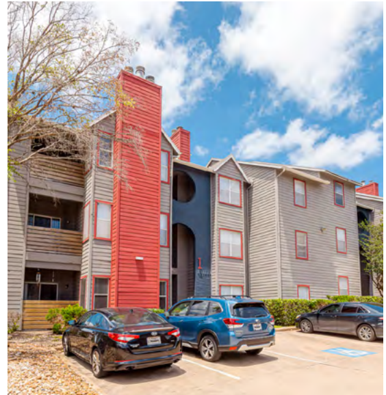
MELROSE TRAIL APARTMENTS: 183 UNITS
