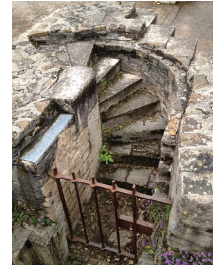
Remains of Spiral Staircase, Cluny (2013)
