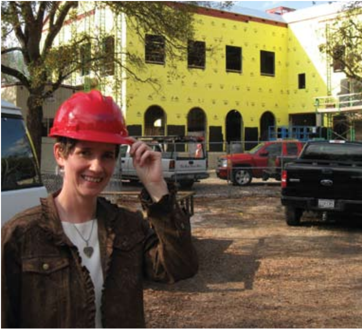
Doretta Fortenberry surveys the progress on Elizabeth Perkins Prothro Hall
